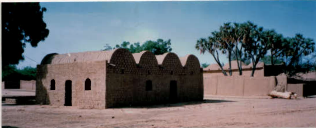
Mosque, Bonkoukou, designed and built by Mallam Abdou.
