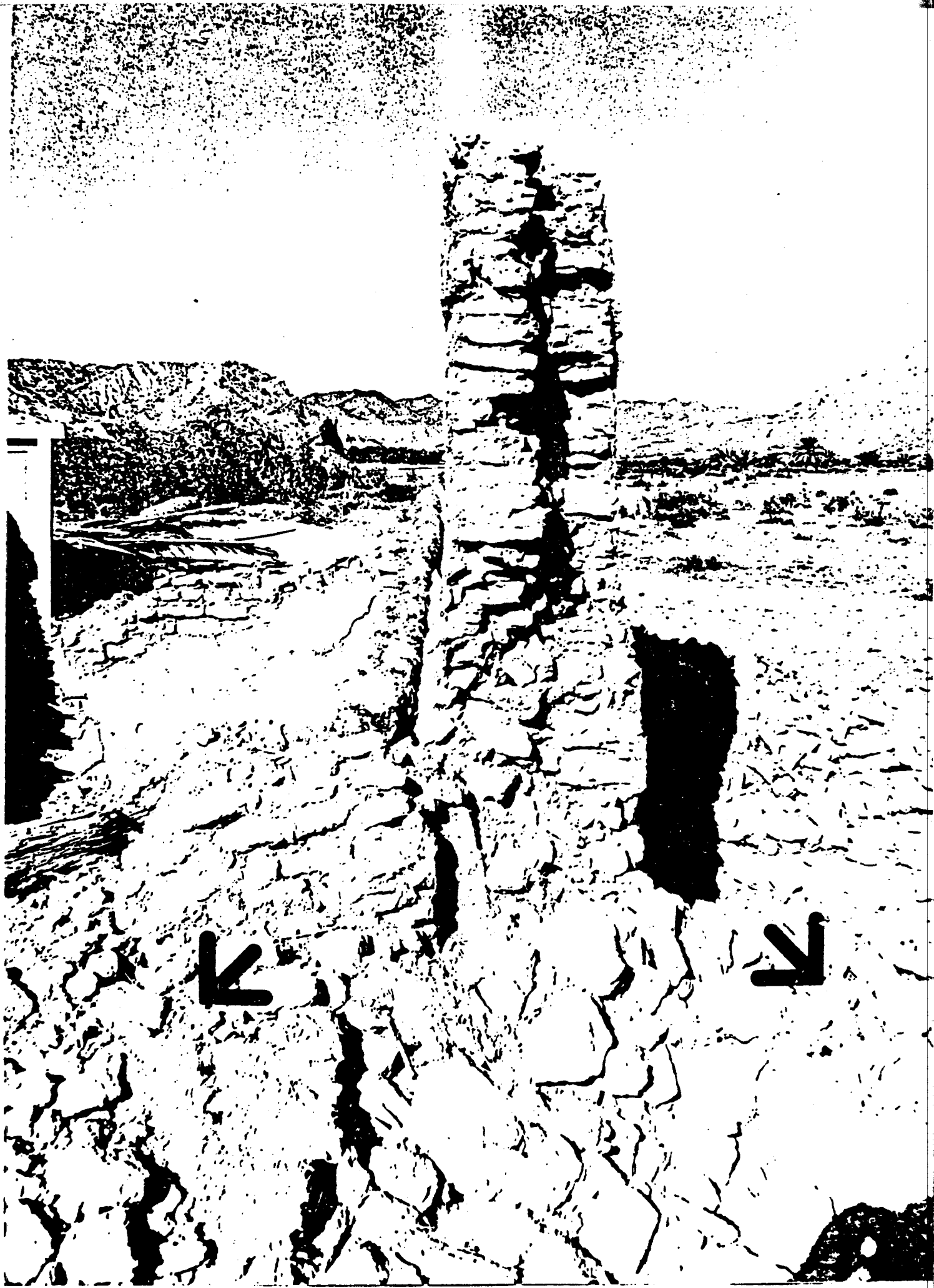
Examples of wall failure due to lack of internal bonding
