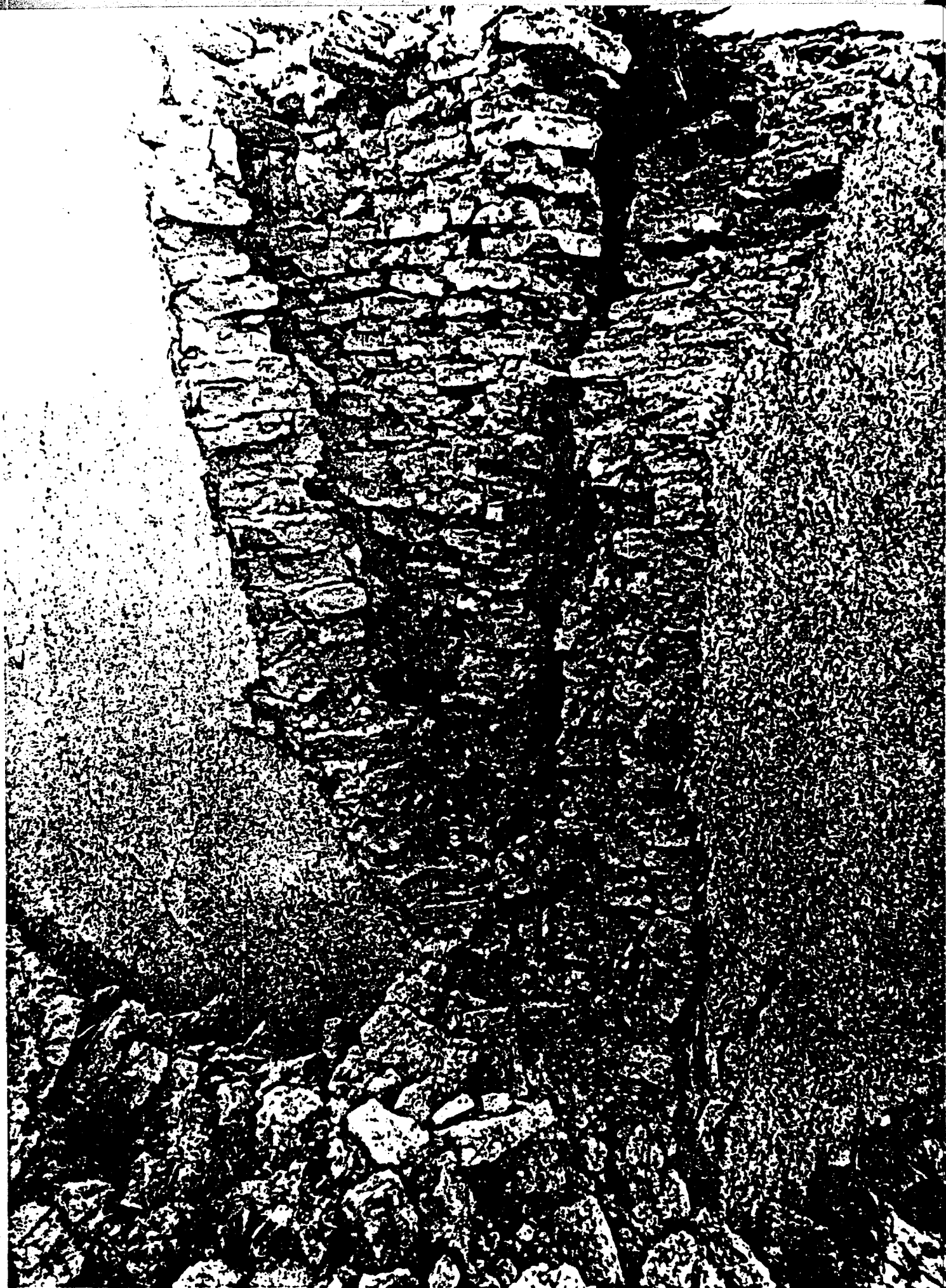
Examples of corner failures - due to stress concentration, poor bonding and lack of reinforcement
