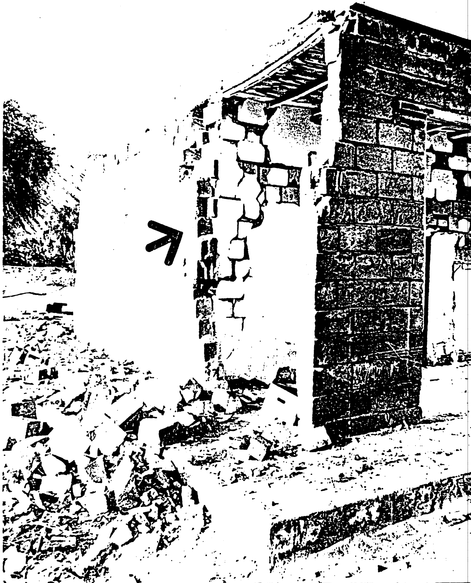
Corner failure and collapse of concrete
