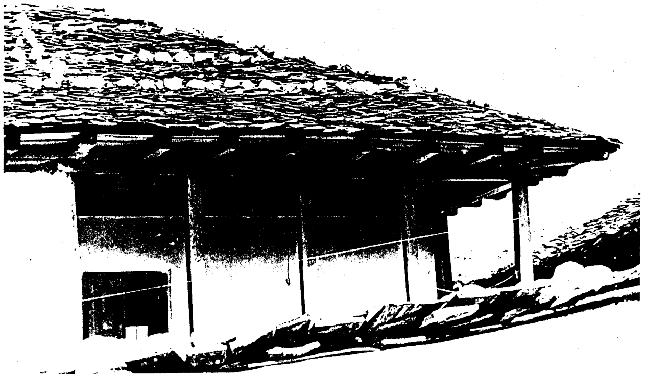
Wood shingles roof. Note stones for weighting down shingles.
