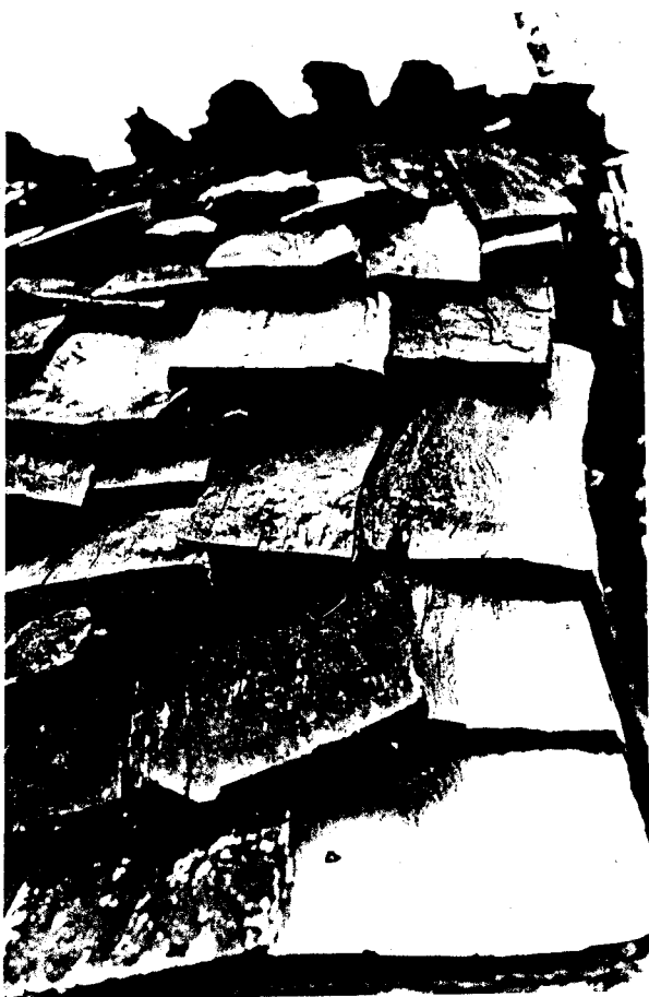
External detail of shingle roof.
