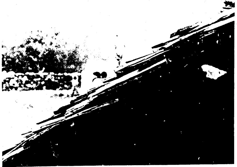
Detail showing overlap of shingles.
