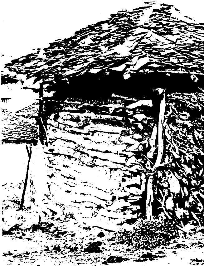
Unrendered log walls are untidy and the mud packing can be washed away.
