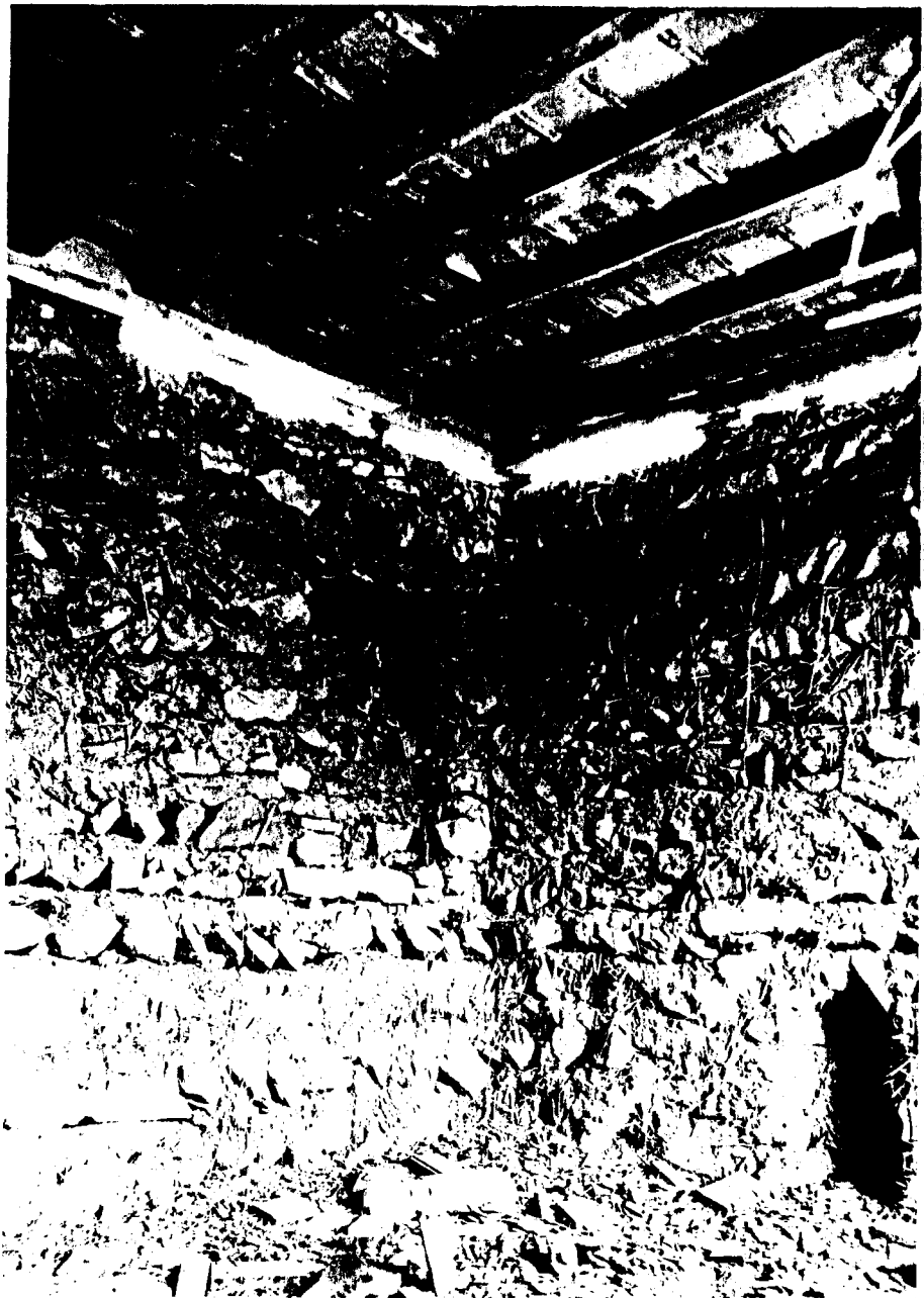
Walls are made of stone and mud. The roof is built as a single framed unit.
