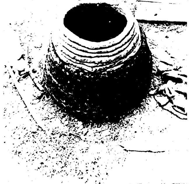
Bread oven being constructed. Clay becomes fired with use.
