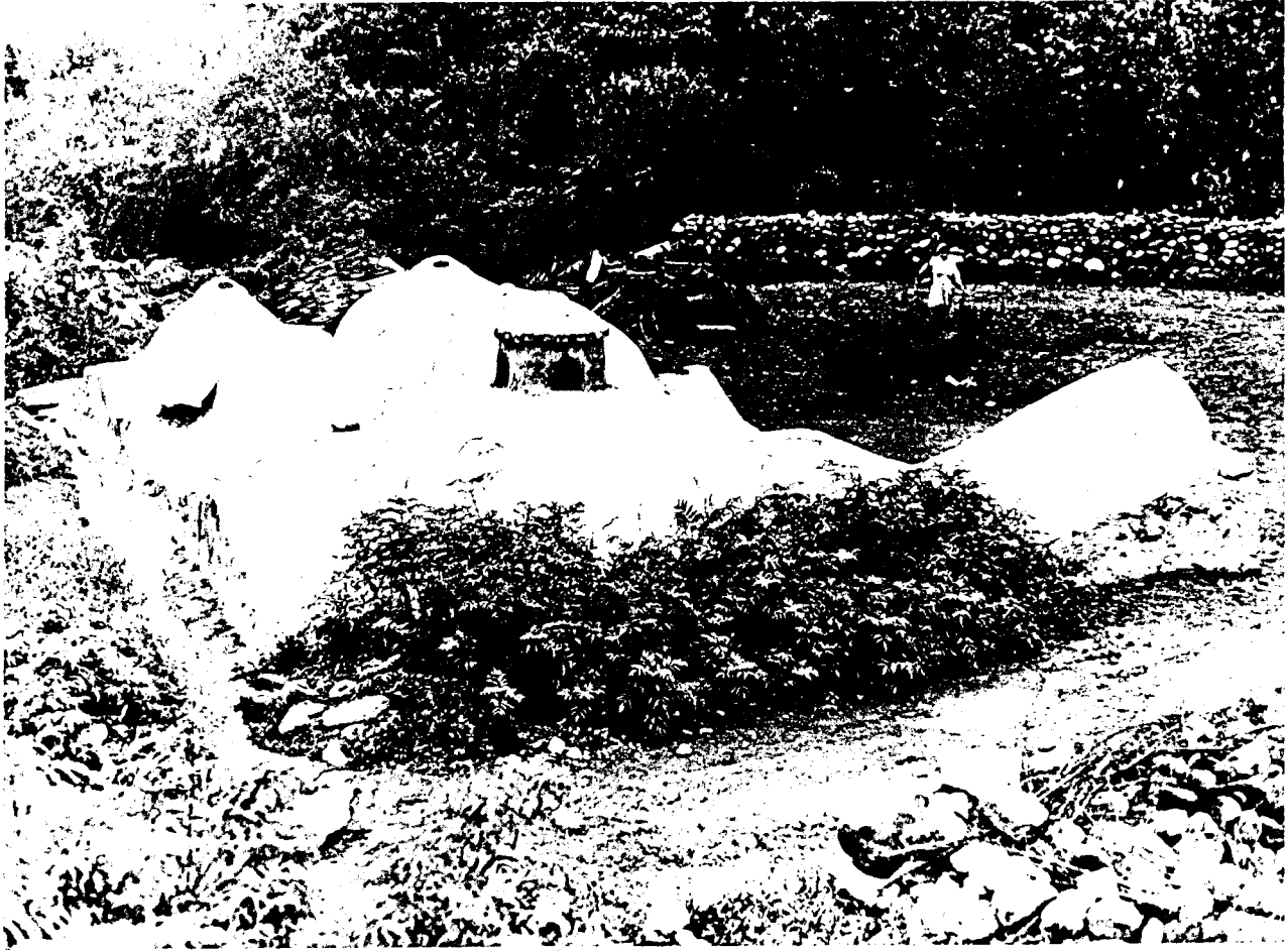
Hamman at Mashalahabad near Abbasabad. Wood fired and relying on gravity controlled water supply.
