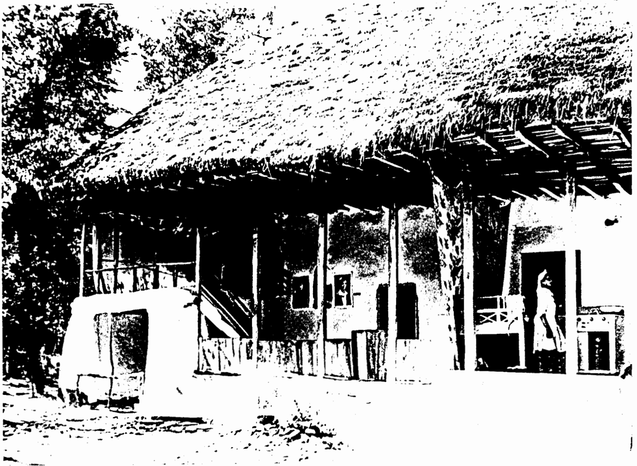
The open platform on the upper mezzanine (the talar) is used for most household activities during warm summer months.
