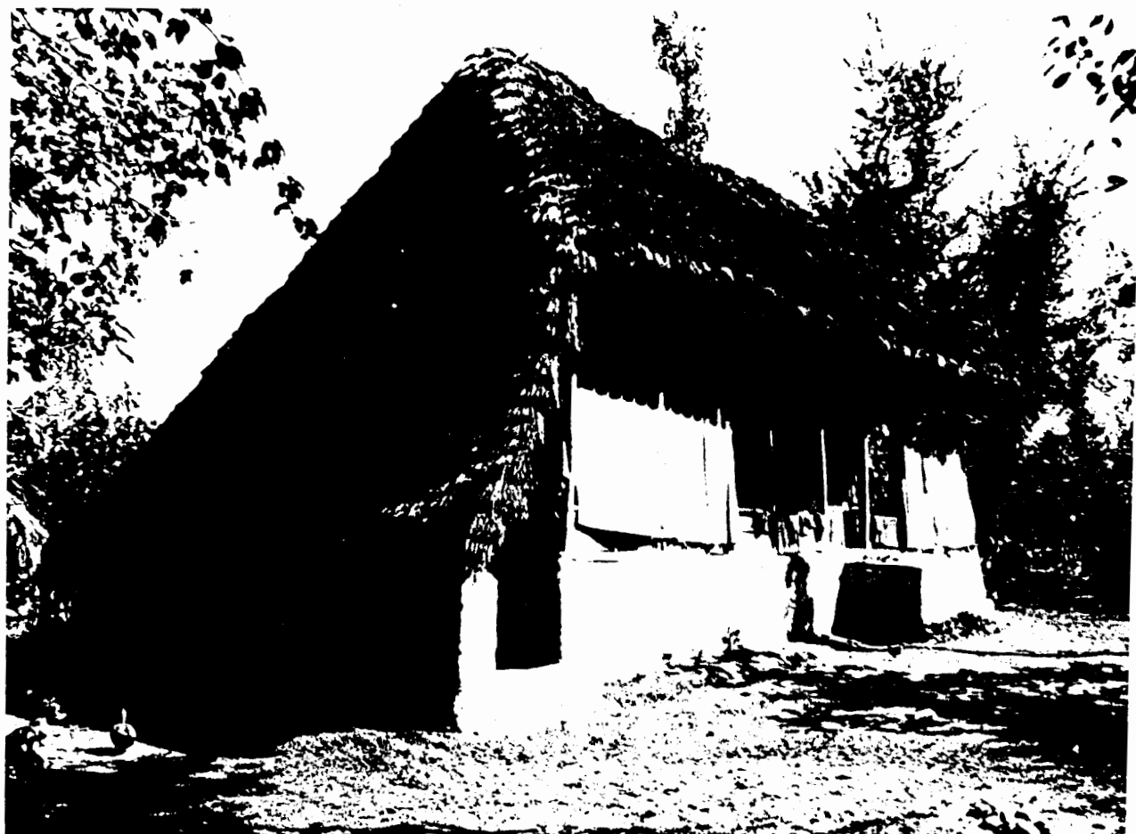
The archetypal two room front aivan house with a protective overhang of the roof eaves in the west side in Dogoor village.
