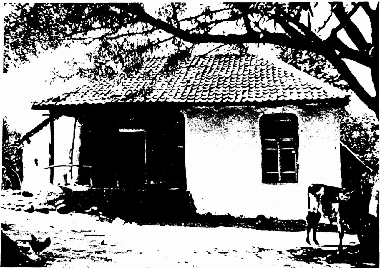
Ancillary shelters are added as lean-to structures to the basic "L" plan house in Kashfi village.
