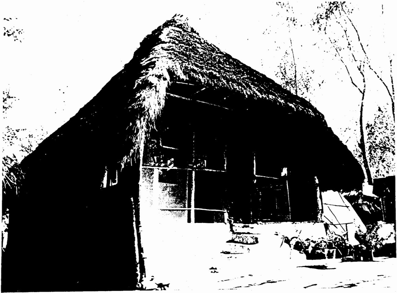
High pitched roofs with the eaves lowered on three sides to protect the walls against high rainfall and winds is a common feature of coastal houses.
