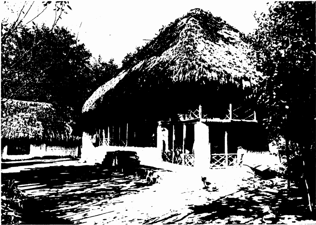
In the rice growing plains settlements a mezzanine (talar) is added to the two room front aivan house.
