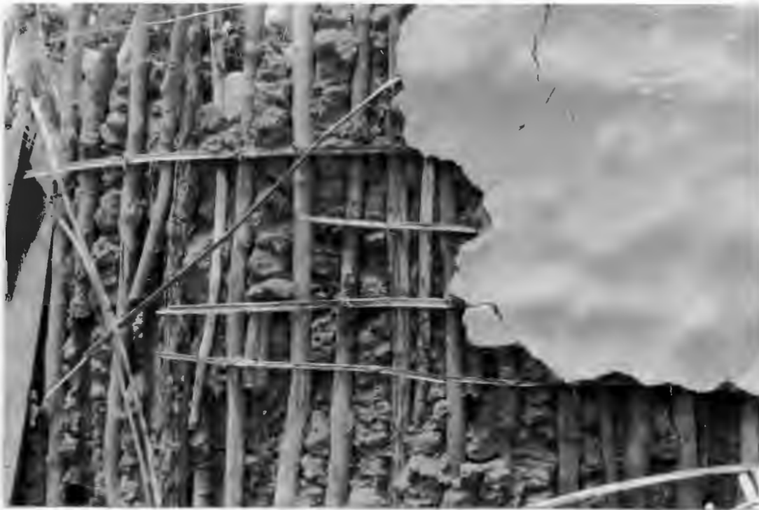
FIG.6. TRADITIONAL WALL WITH WOOD AND BAMBOO FRAME COVERED BY MUD PLASTER
