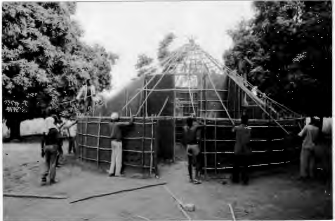
ROOF FRAME IN POSITION ON WALLS. ROUND HOUSE.
