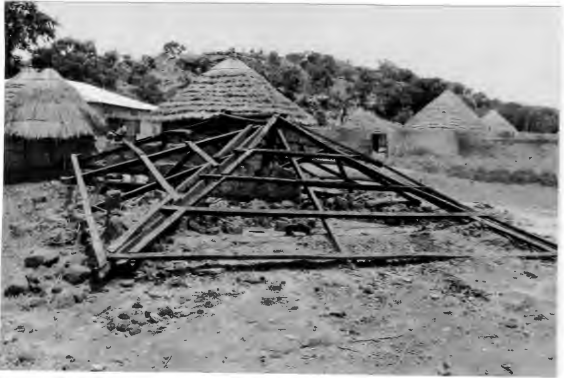
FIG. 12. RECTANGULAR HOUSE ROOF FRAME RESTING ON RUBBLE OF COLLAPSED WALLS. KOUMBIA
