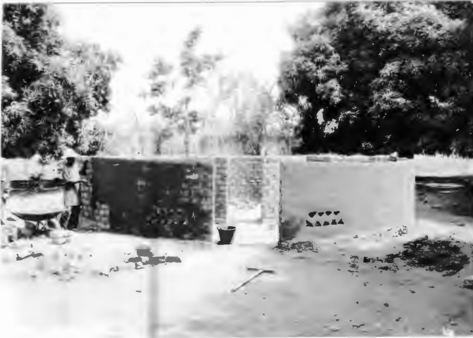
A). ROUND HOUSE OUTER WALL BEING PLASTERED (AT MADINA GUILLEDJI).
