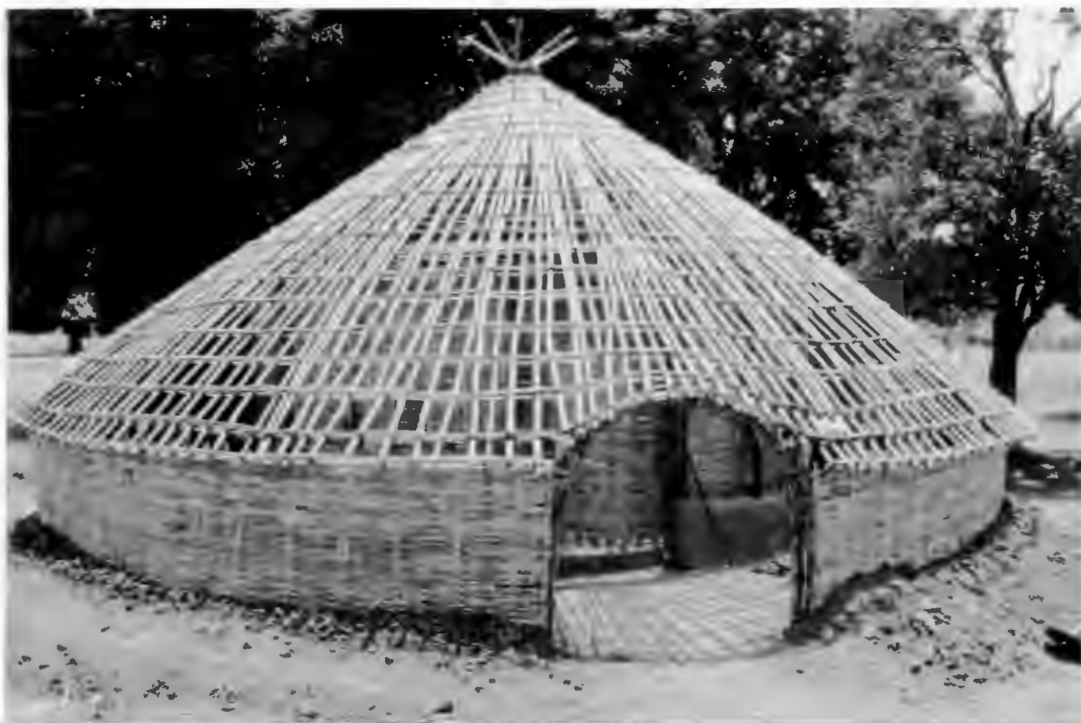
FIG.7. ROOF FRAME READY FOR THATCHING ON TEMPORARY HOUSE NEAR KAMELE
