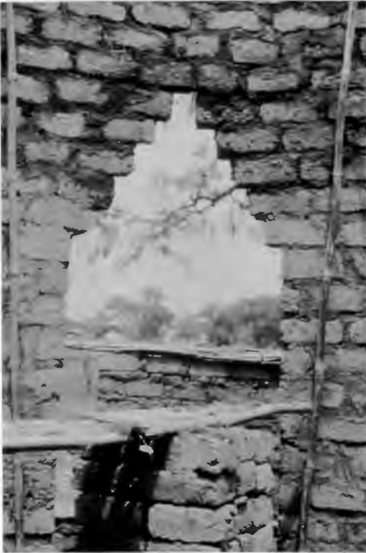
FIG. 21. CORBEL ARCH OVER OPENING, INNER CIRCLE WALL OF ROUND HOUSE. VERTICAL BAMBOOS ALREADY IN PLACE.
