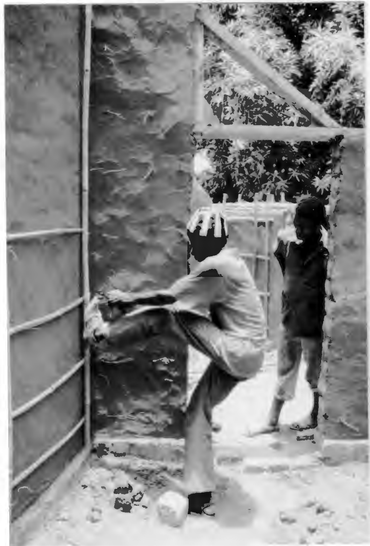
C). PUSHING THE FRAMES AGAINST THE WALL. VIEW LOOKING DOWN.
