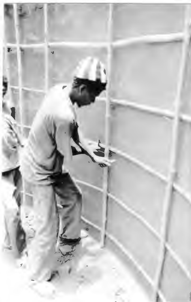
F). BINDING THE WIRES USING STICKS
