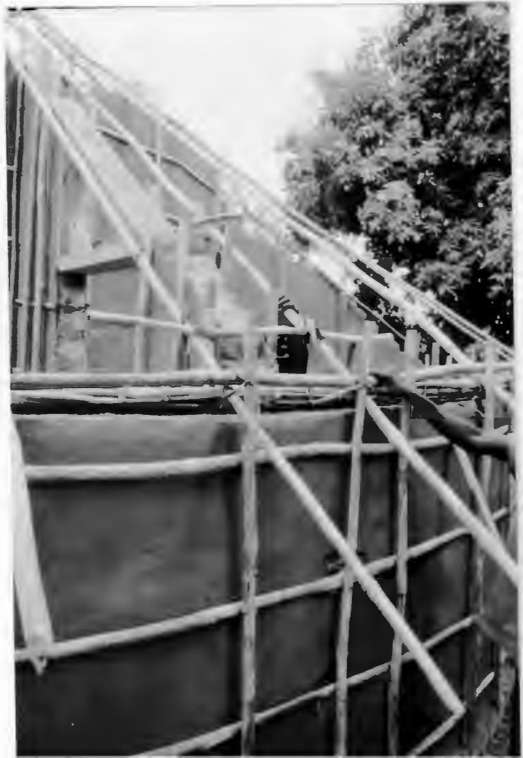
ROOF FRAME ATTACHED TO WALL FRAME.
