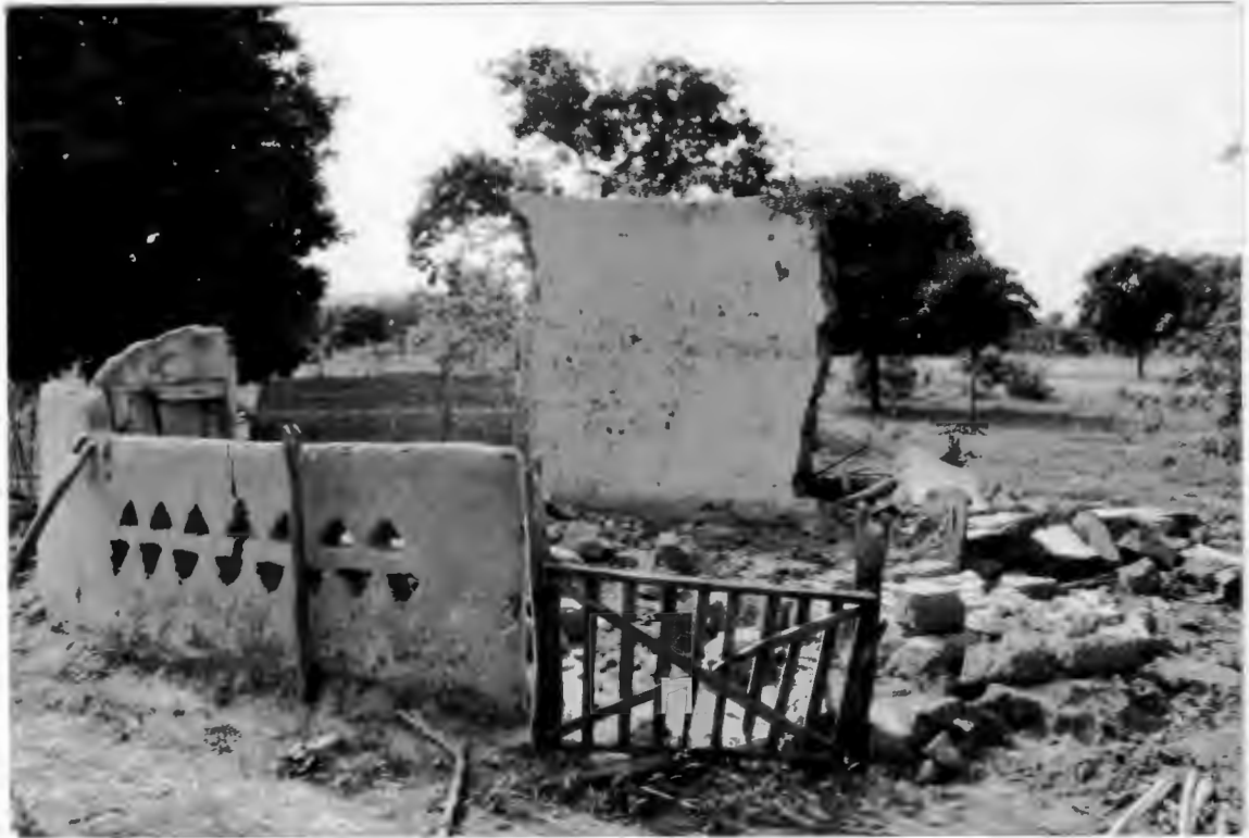
FIG.10. TALL SEGMENT OF WALL REMAINING ON ROUND HOUSE INNER WALL, AFTER COLLAPSE OF LINTEL AND MOST OF INNER WALL.
