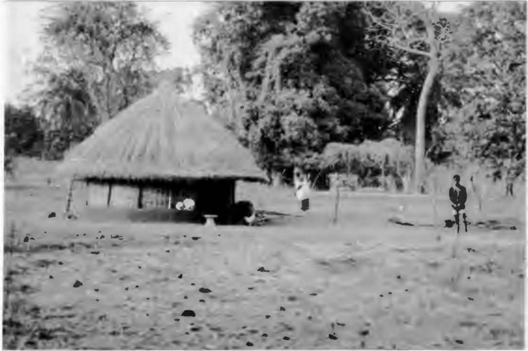
TEMPORARY ROUND HOUSES WITH BAMBOO MATTING WALLS.
