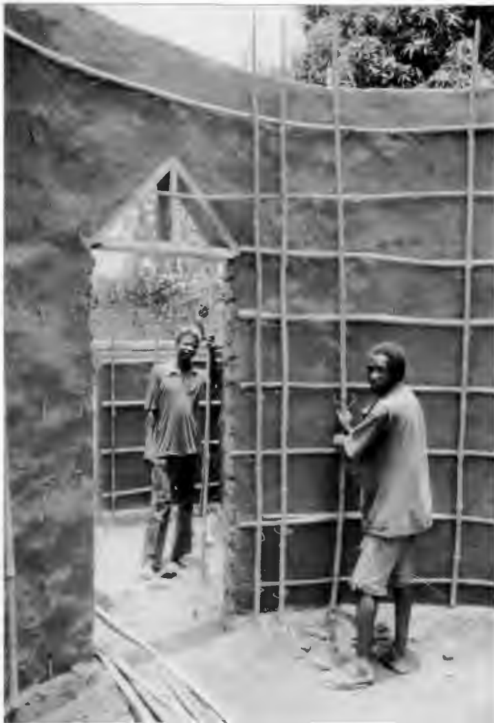
A). ROUND HOUSE OUTER WALL BEING PLASTERED (AT MADINA GUILLEDJI).
