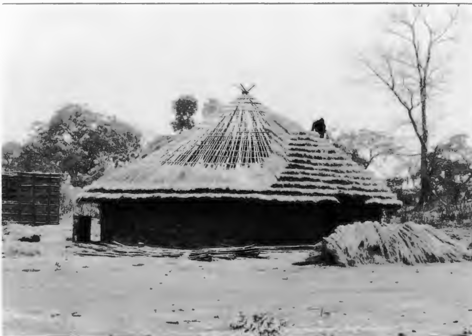
FIG. 39. THATCHING THE ROOF
