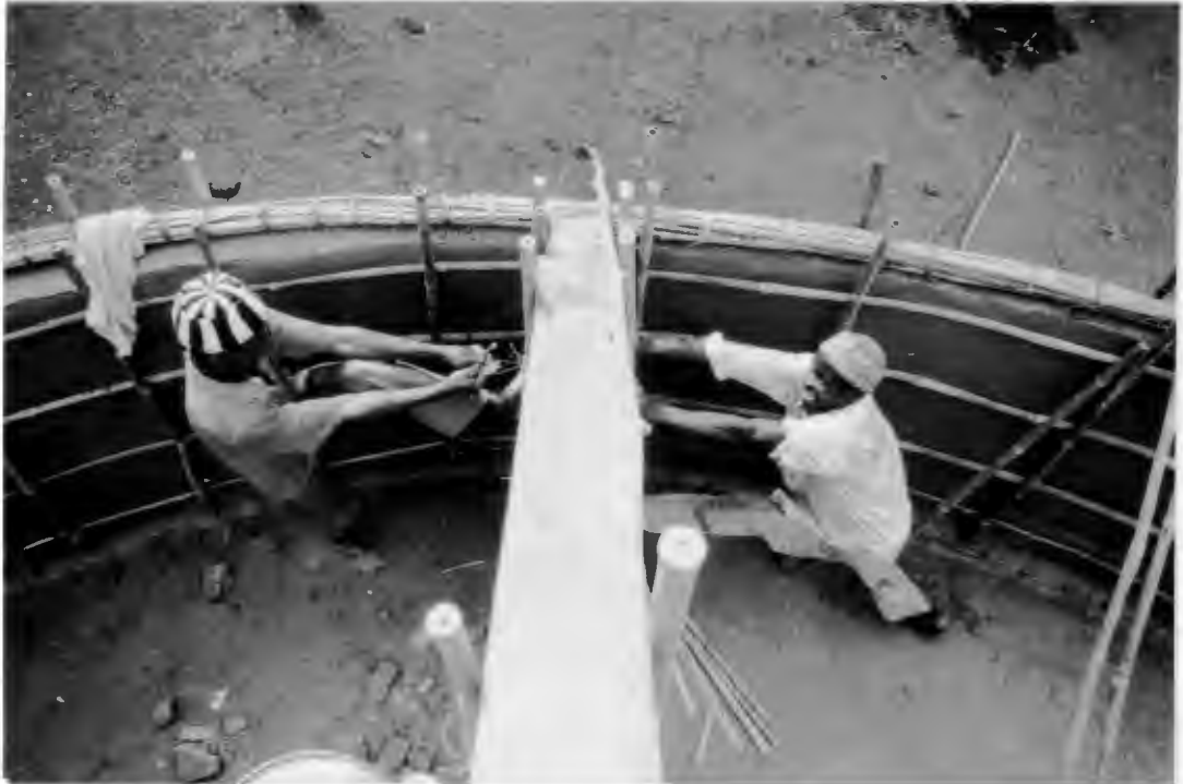
C). PUSHING THE FRAMES AGAINST THE WALL. VIEW LOOKING DOWN.
