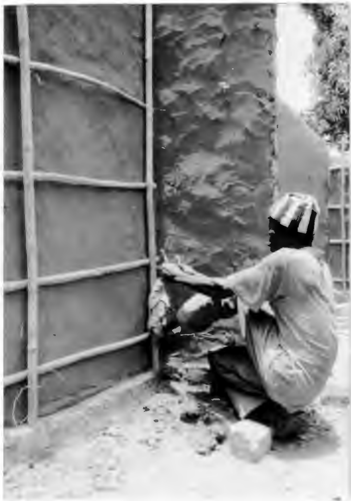
E). PULLING WIRES TIGHT
