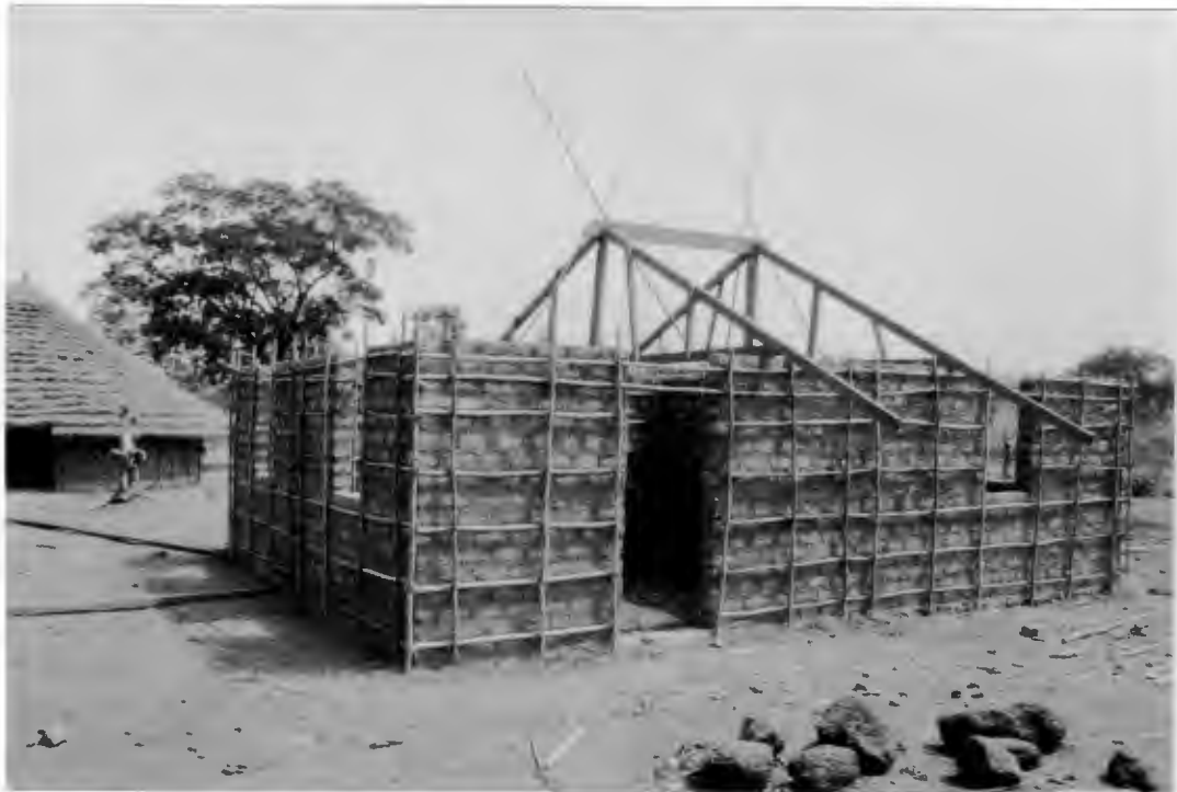
DEMONSTRATION RECTANGULAR HOUSE (LOCAL MATERIALS) READY FOR ROOFING.
