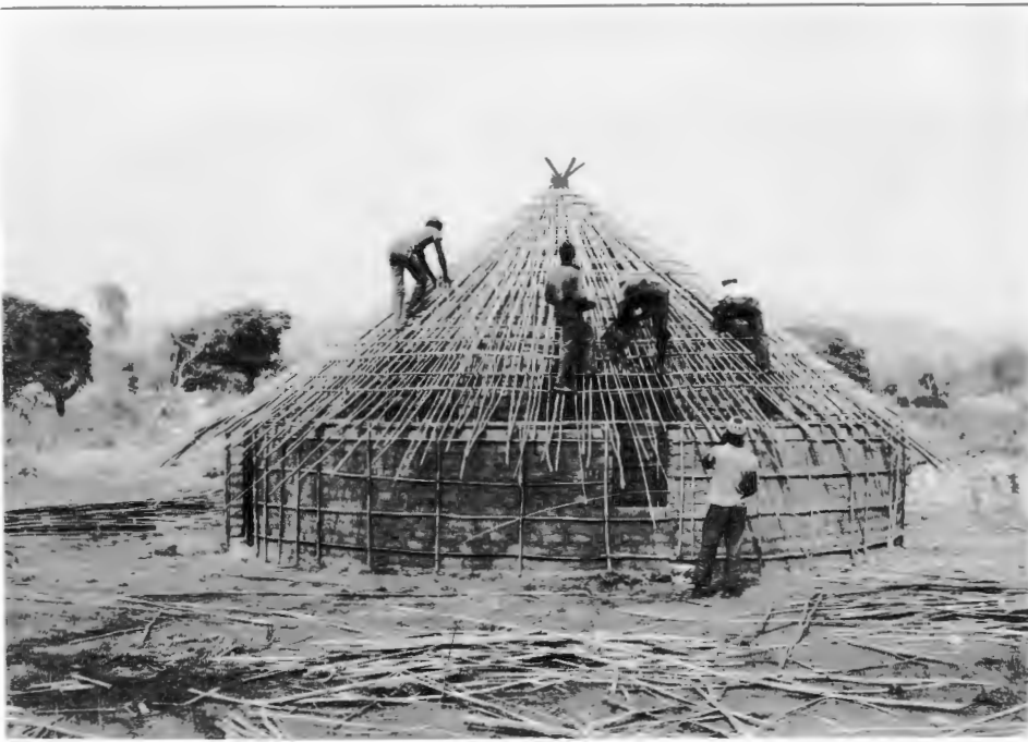
FIG. 38. ADDITIONAL HORIZONTAL BAMBOO RINGS BEING PLACED ON ROOF FRAME
