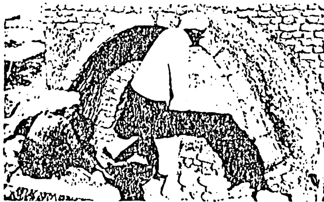
Because of the adhesiveness between mud brick and mud mortar Domes and vaults can be built without any supporting framework.
