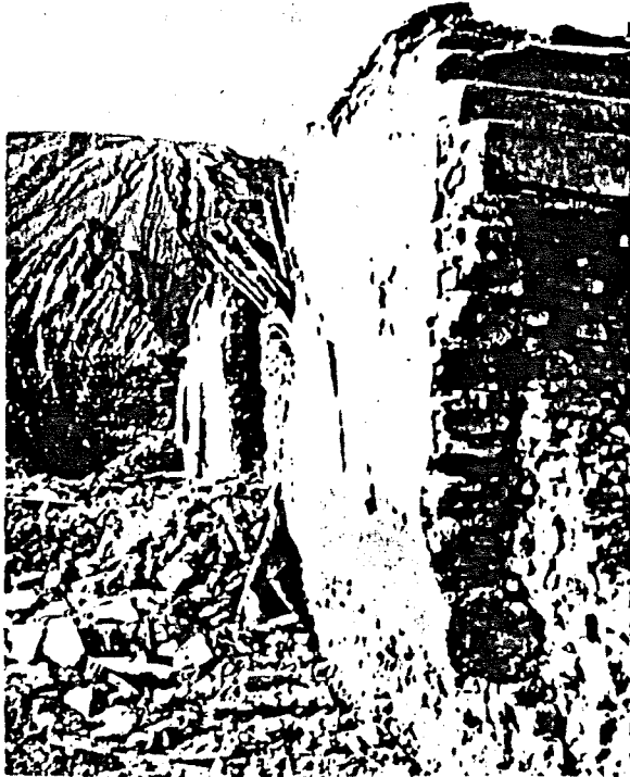
Examples of wall failure due to lack of internal bonding
