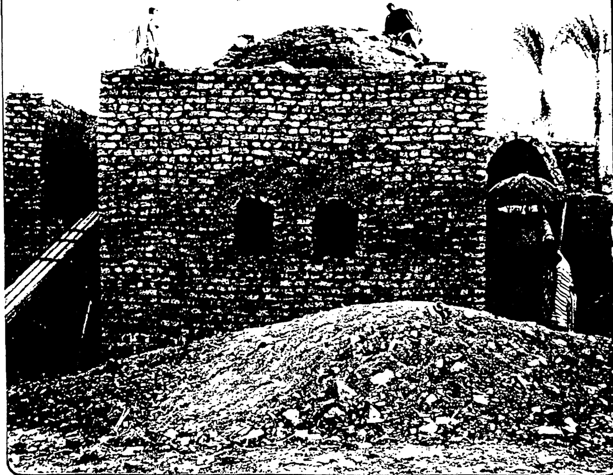
Vault building with centers leaving inward and out wall so that no firm work or shoring is needed.
