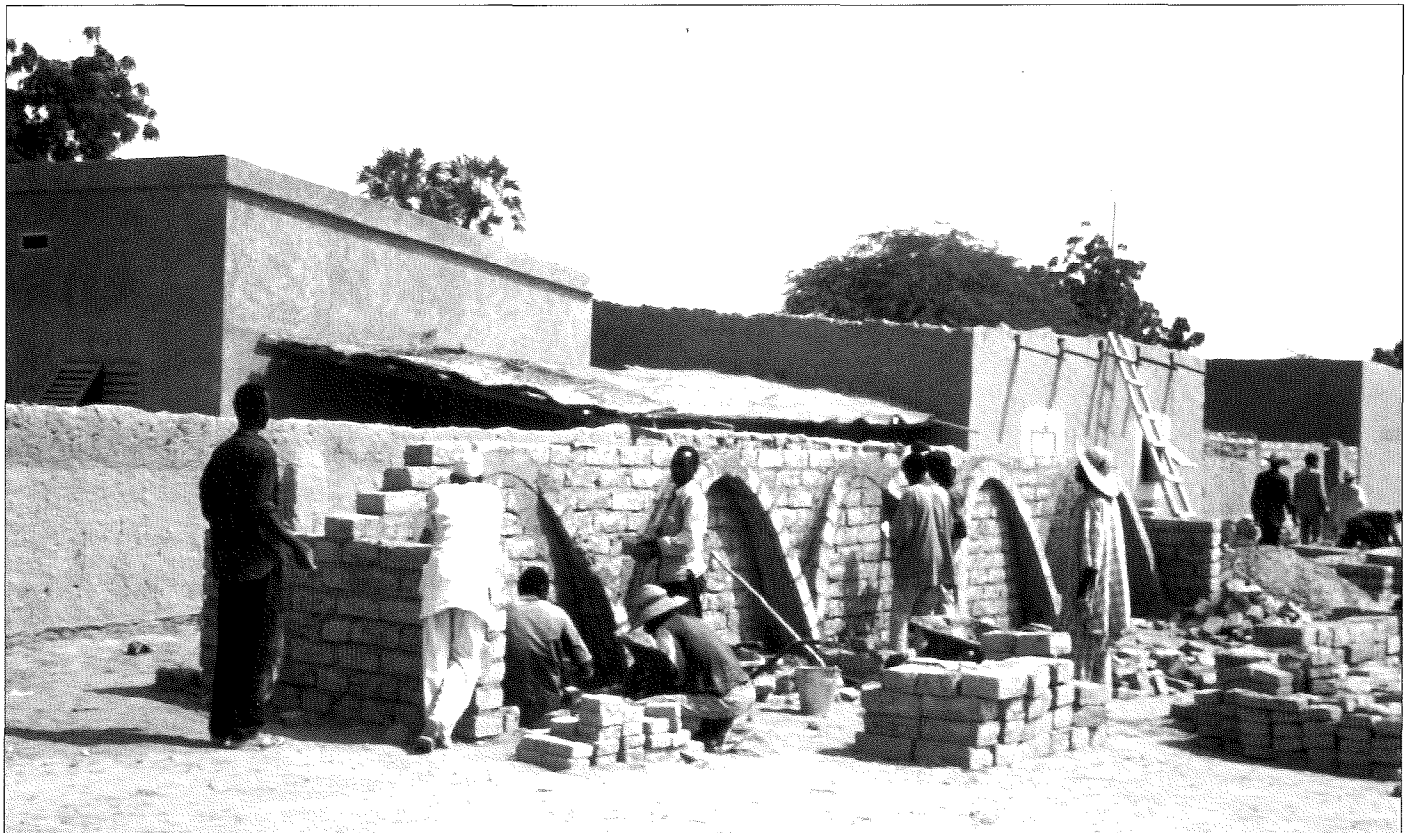
Fig. 1. Training of trainers and builders in woodless construction techniques (vol. 2)
