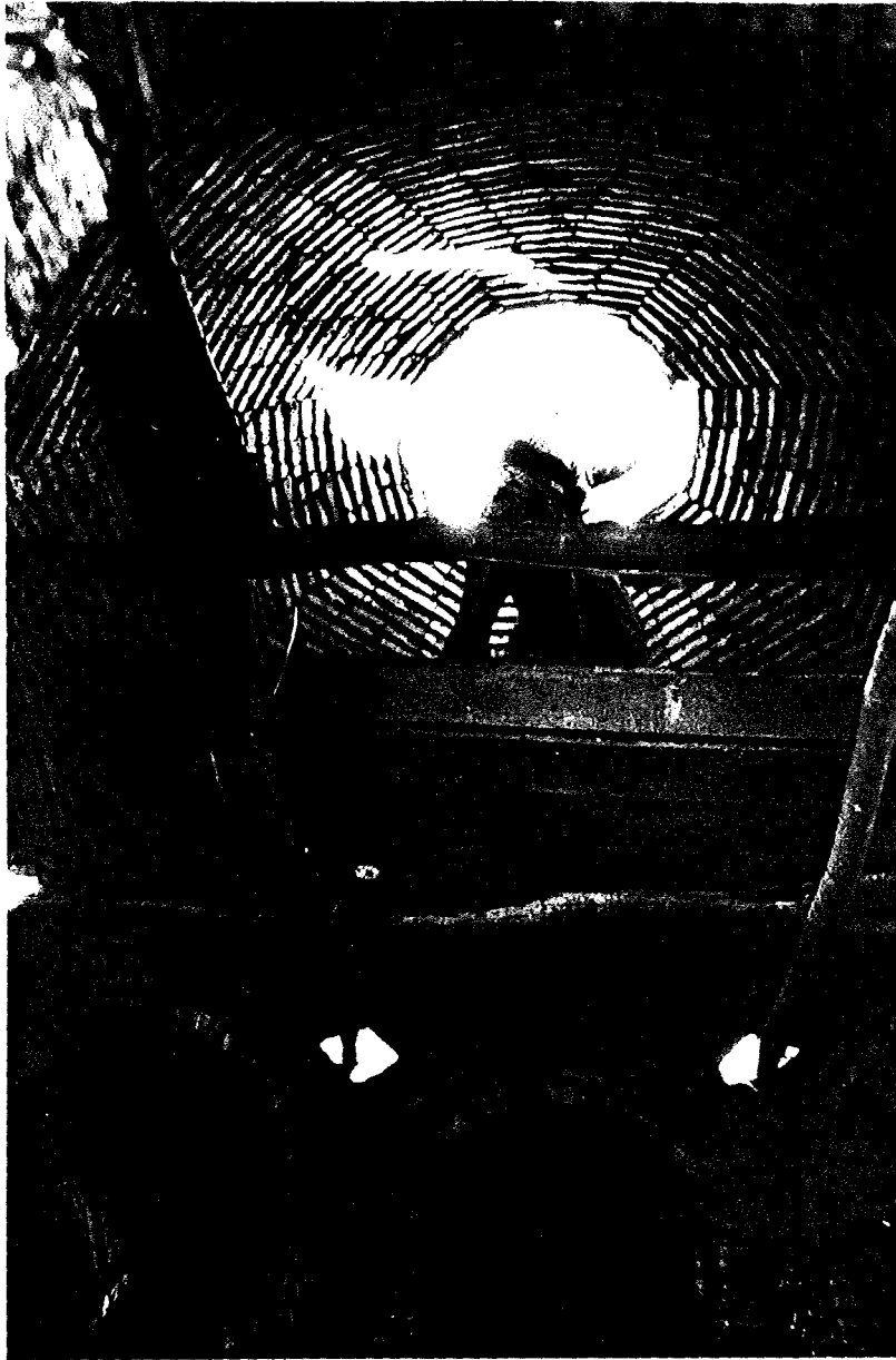
Dome construction over shower room Niazabad Hamman SIDP Iran.
