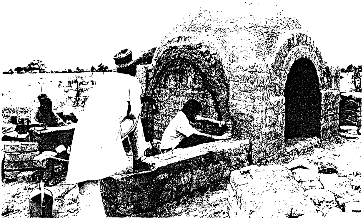
Literacy Centre, Chikal, Niger Training local builders in vault and dome ^ technology.
