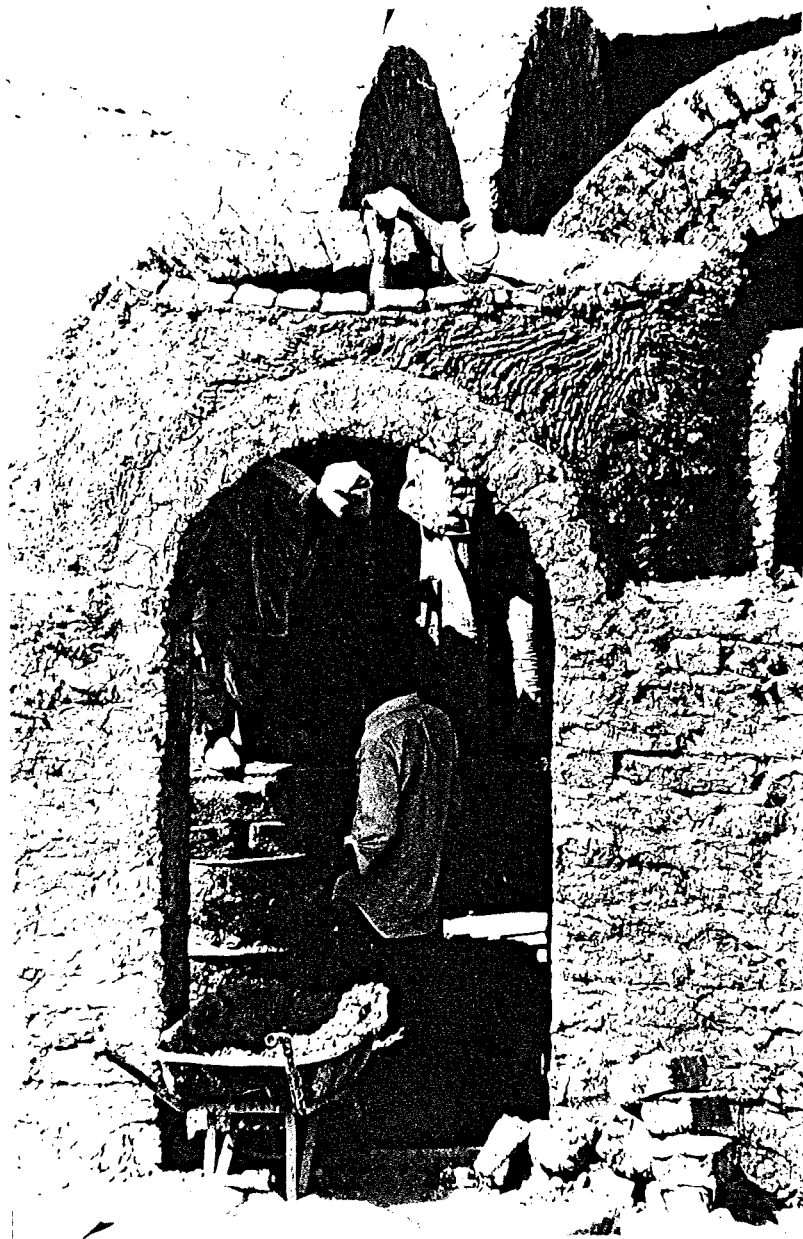
Literacy Centre, Chikal, Niger Construction of dome over entrance
