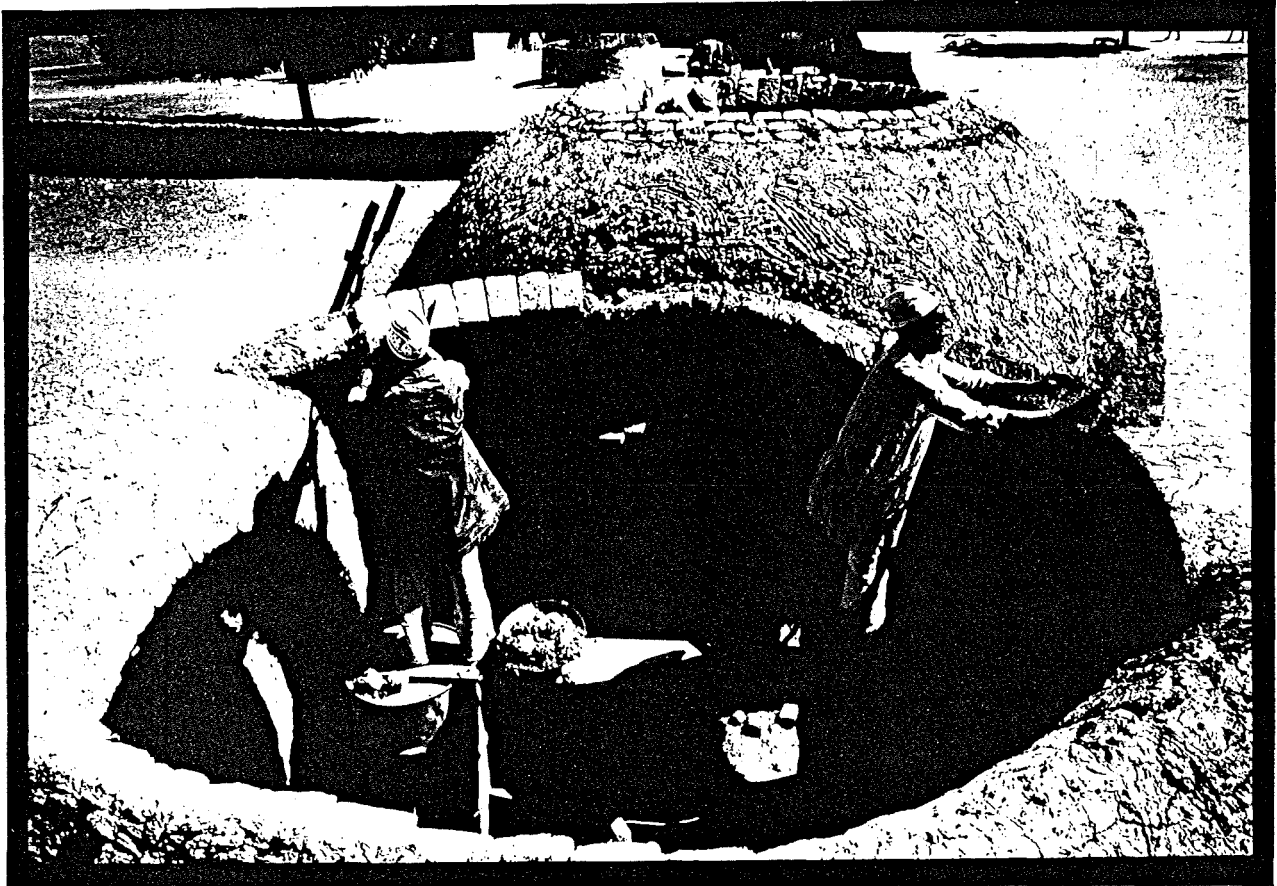
Literacy Centre, Chikal, Niger Construction of Dome over classroom ^
