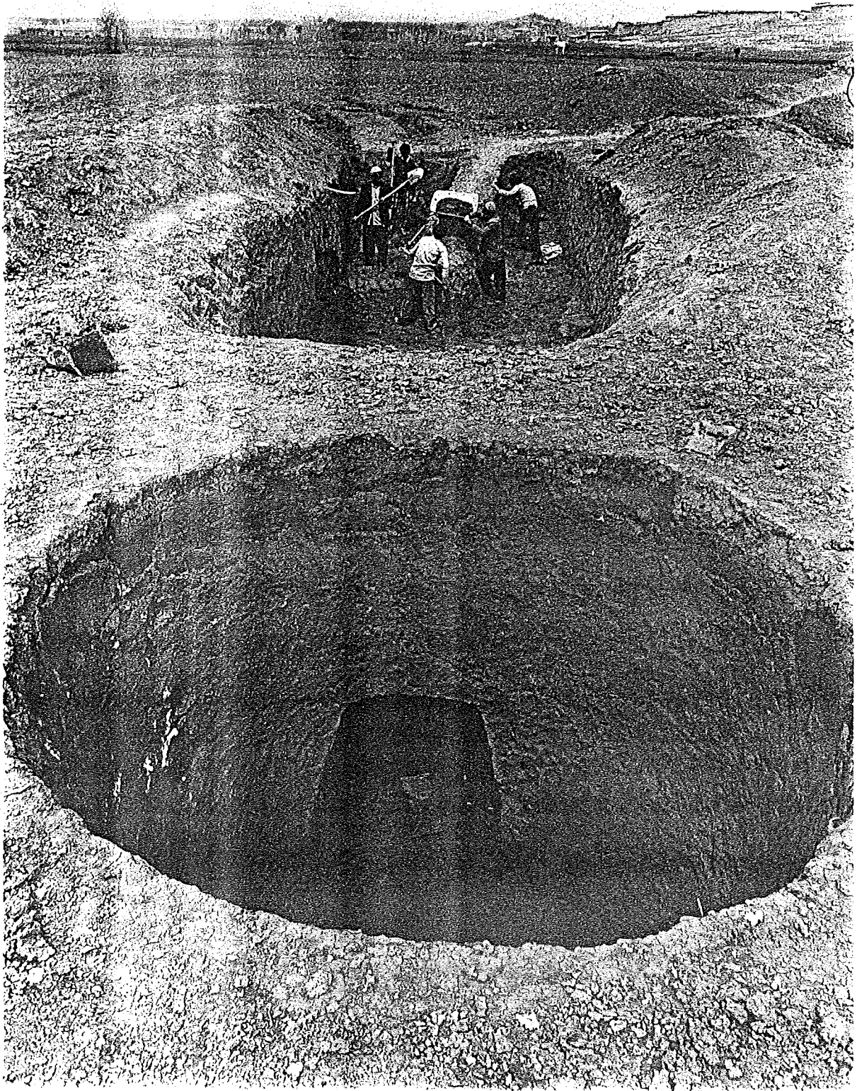
Brick and lime kiln under construction at Kamar Siah. SIDP. Iran.
