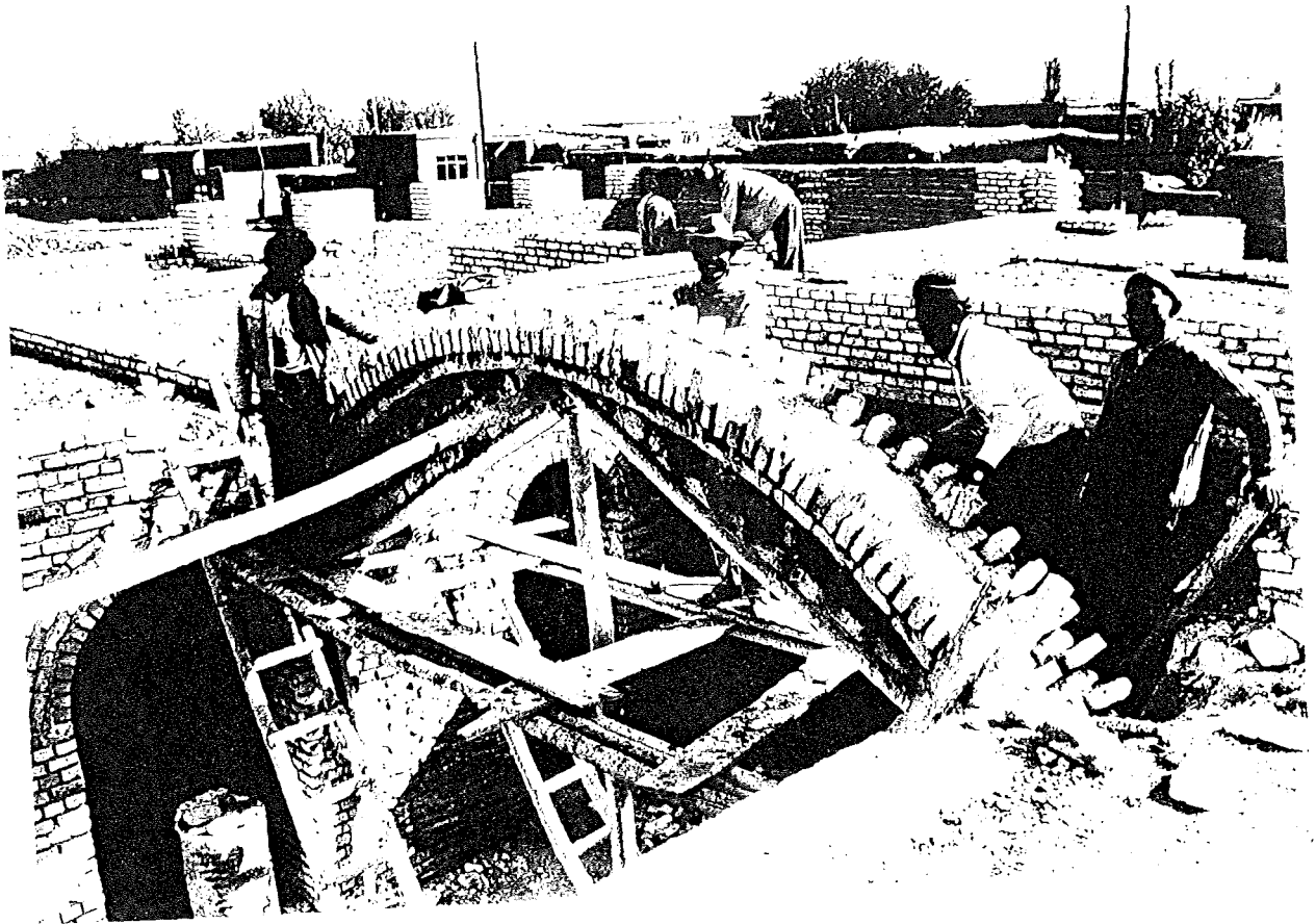
Construction of Arch across 7m wide classroom Alashtar Kindergarten SIDP Iran
