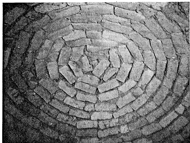
dome built of unstabilized mud brick - requiring no wood ...
