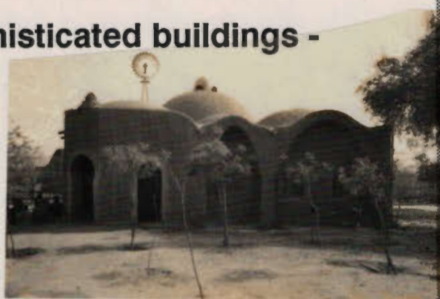
project office building (Chikal, Niger).
