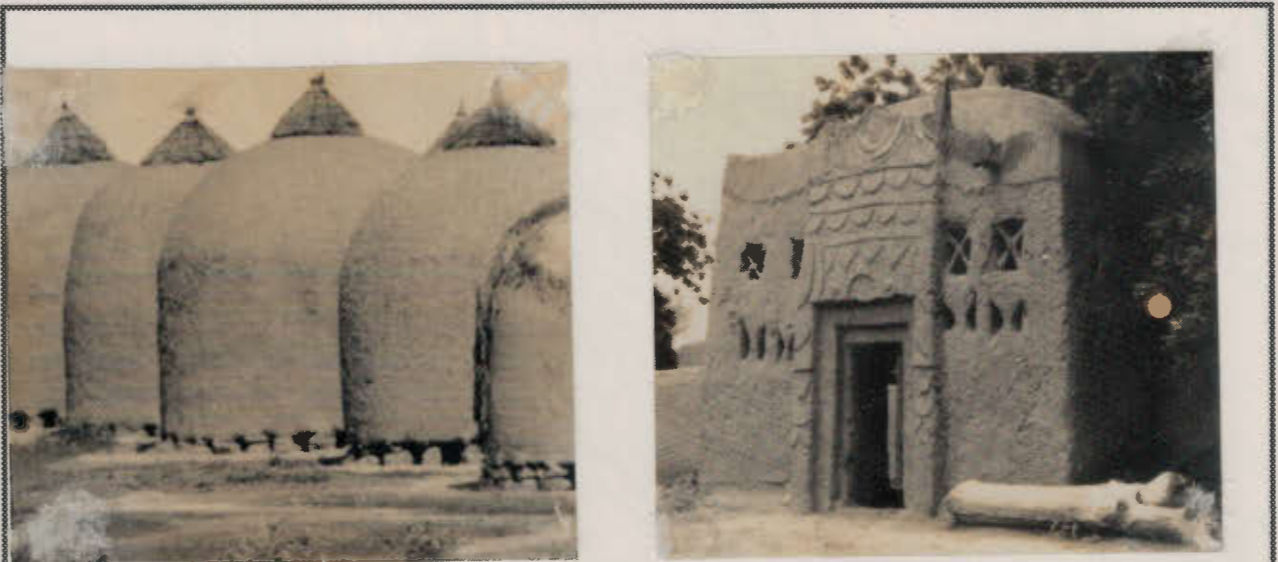
domes are a familiar sight throughout the Sahel, particularly on the thin "coiled" walls of granaries...
