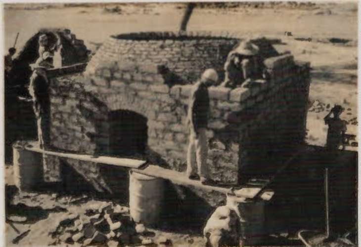
woodless construction of a small rectangular domed shelter (Niger) -
