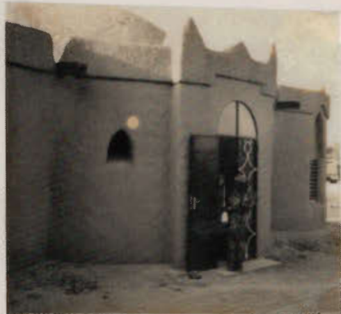
crafts centre in Agadez (Niger): simple structure with good quality finishings
