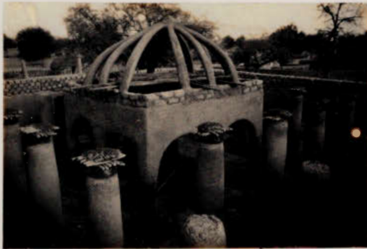
'traditional' construction of a mosque (Niger) -
