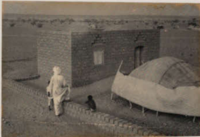
two-room domed house built by mason for his own family with no external financial or technical support (Tchlozerine, Niger).
