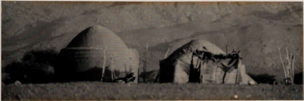
simple round domed shelter, built entirely from unstabilized mud bricks; its shape is reminiscent of that of the traditional tent (éhan) built from organic materials...
