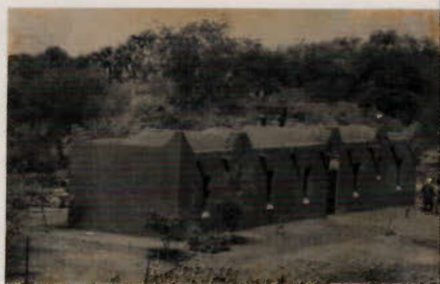
vault and dome communal housing (Catholic Mission, Tchirozerine, Niger).
