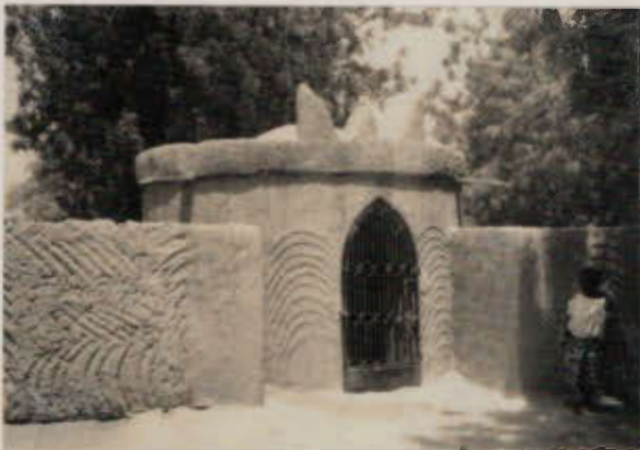
a traditional decorative render gives this small building "local colour" (Dosso, Niger).
