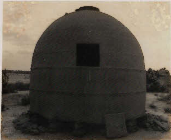
"Coil" construction granary typical of many regions of the Sahel, with thin unstabilized earth walls. Local knowledge of how to ensure that such buildings resist heavy downpours of rain exists...
