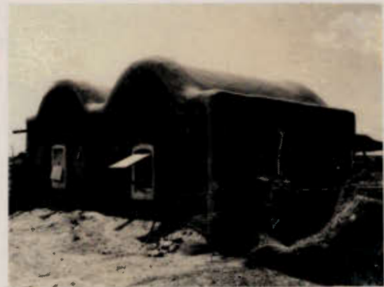
unusually, here the poor quality of the local soil justified a small addition of cement to the roof and the most exposed façade.
