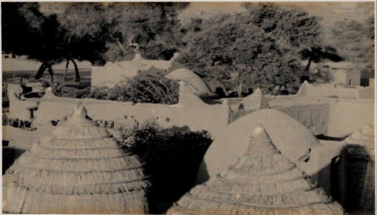
a changing roovescape - woodless vaults and domes alongside "traditional" flat roofs (with wooden beams) and straw huts in Iférouane, (Niger)
