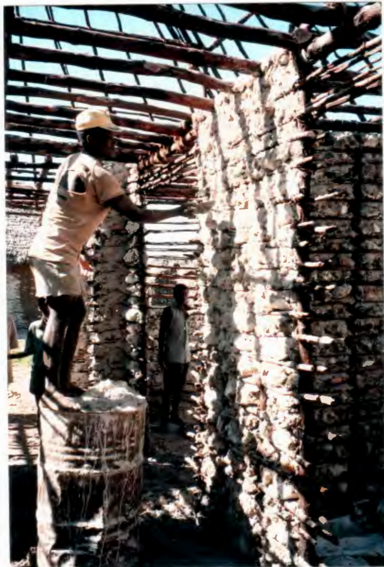
Wall building on Jibondo
