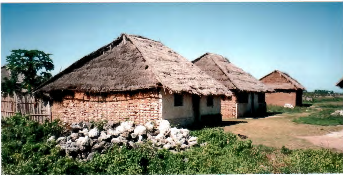
Houses at different stages of completion on Jobondo
