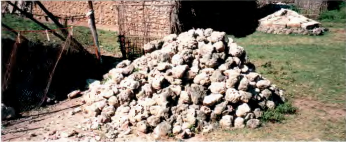
Coral lumps ready for facing an existing house, Jibondo
