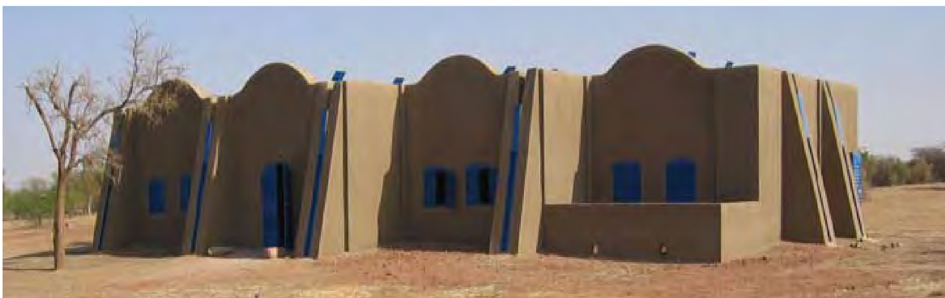
Oursi Beero museum, built with woodless construction (mud bricks, vaults, local renders) in northern Burkina Faso
