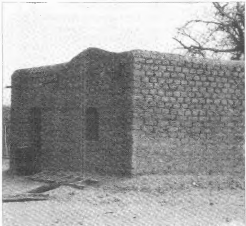
Completed soon after Mr Ly sent his article, the first house built without wood in Loboudou village.
