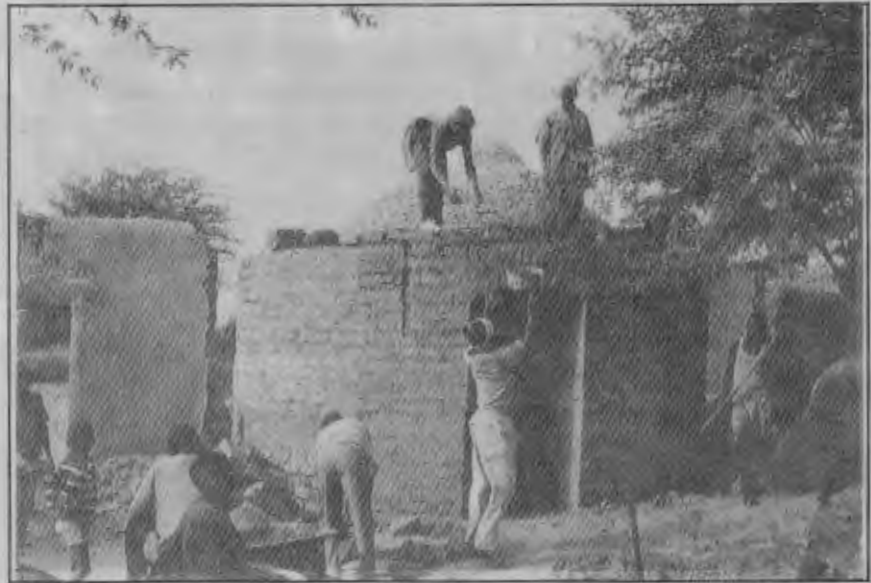
A Dome being built in Mali as woodless construction
