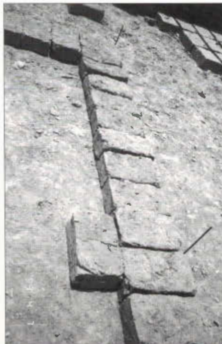
Figure 1 Ordinary mud bricks of local dimensions are used as the unit of measurement in laying out. Increasingly only header courses are used.
