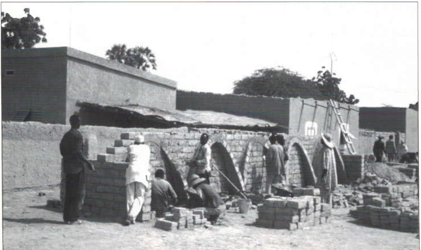
Figure 1 Trainee masons practice starting off vaults on training structures (phase 2)
