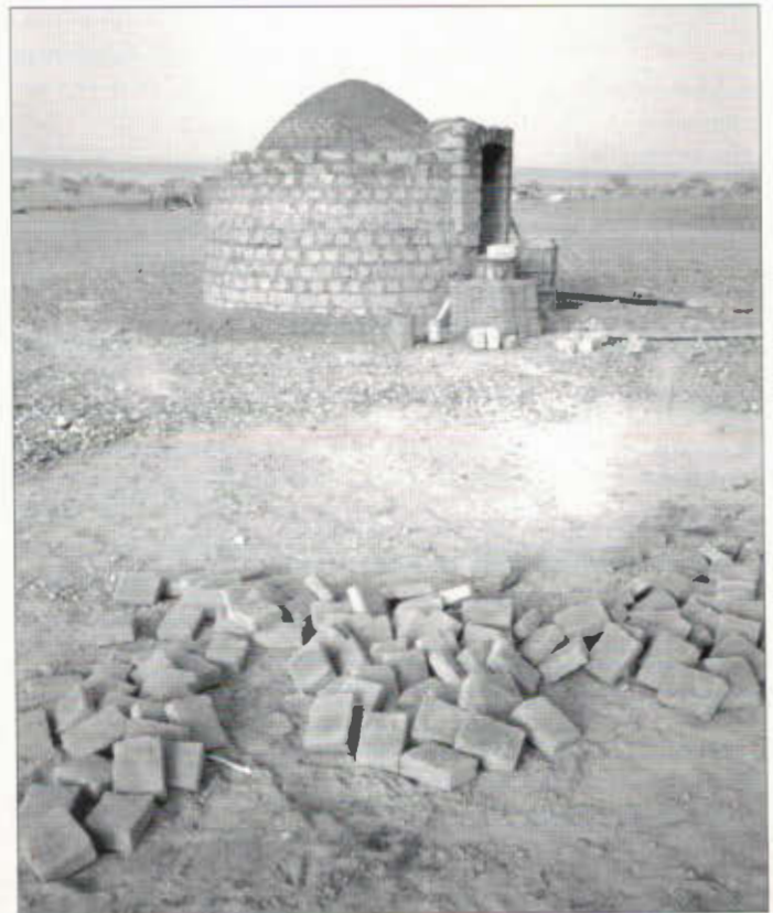
Figure 2 Round dome structure – a cheap, easily built shelter
