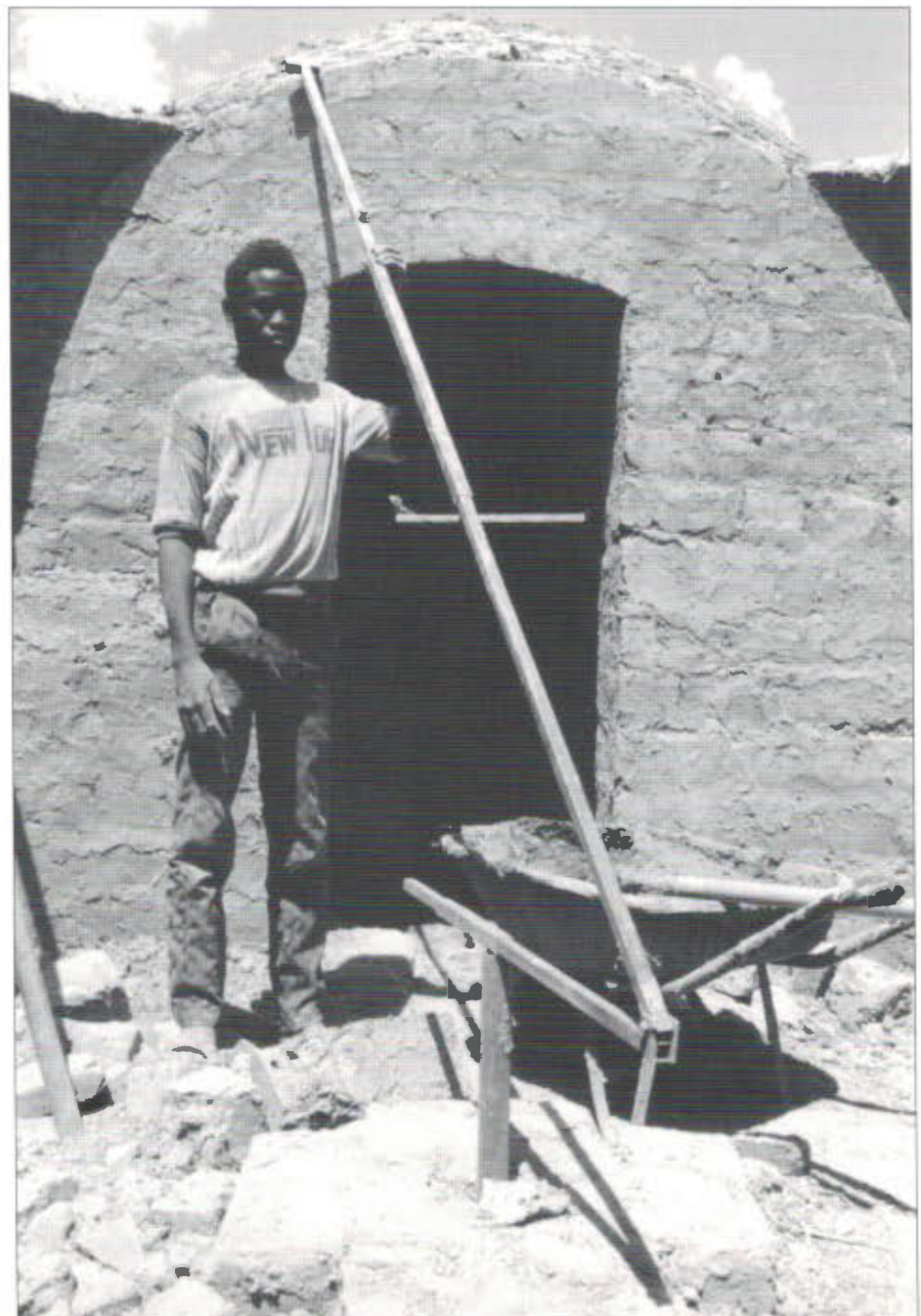
Figure 3 An adjustable radial arm is given to each mason at the end of his basic training, enabling him to build eccentric domes.
