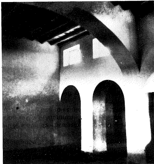
Methods developed to increase spans of local timber for classroom use.
